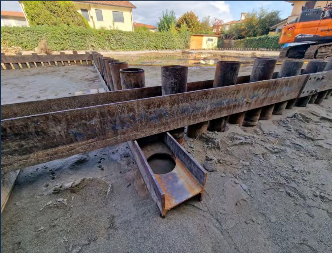
The **Geonord wellpoint® Waterjet Modular Wall** allows the most varied combination of installations, is possible:
