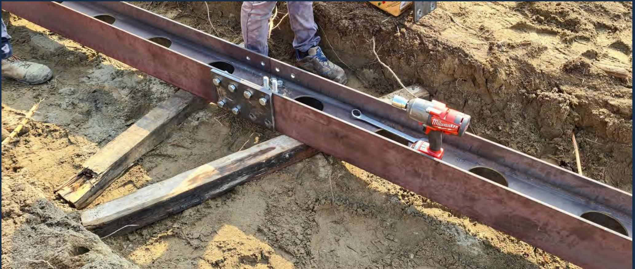
The head beams, suitably pre-drilled, allow a modular type assembly of the piling.
