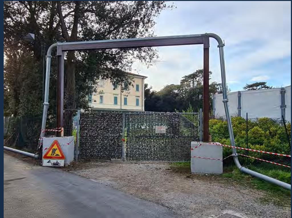
**Geonord wellpoint®** rents various preparatory equipment for the installation of pipes for pumping systems, among these we find the **Mobile Road Portals**.
