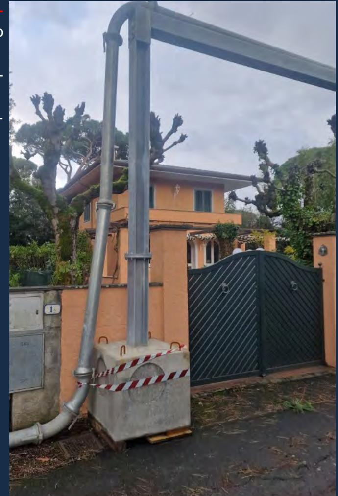
The jamb consist of **HEA200** type S355 steel profiles and can be rented both in the **single pillar solution** with a height of 455 cm., and in the **variable height version**, with flanged upright fixed in the base and counter-flanged upright in the elevated part.
